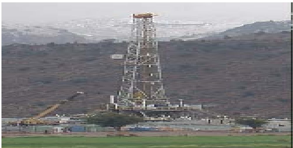
Drilling in Progress –Tal Block
